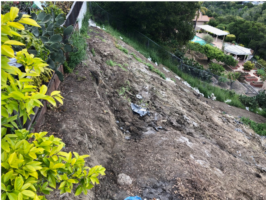
Photo 3: View towards the northeast of the top (head-scarp area) of the affected portion of the slope.
