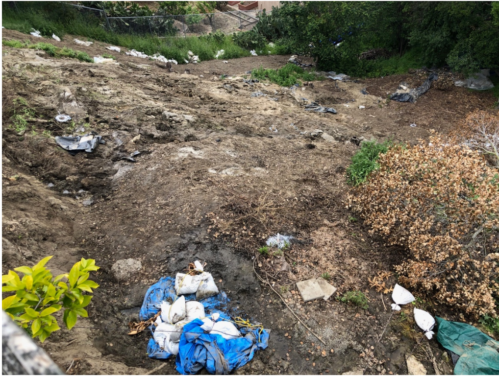
Photo 2: View towards the east from the wooden porch behind 2843 Arguello of the slide area.
